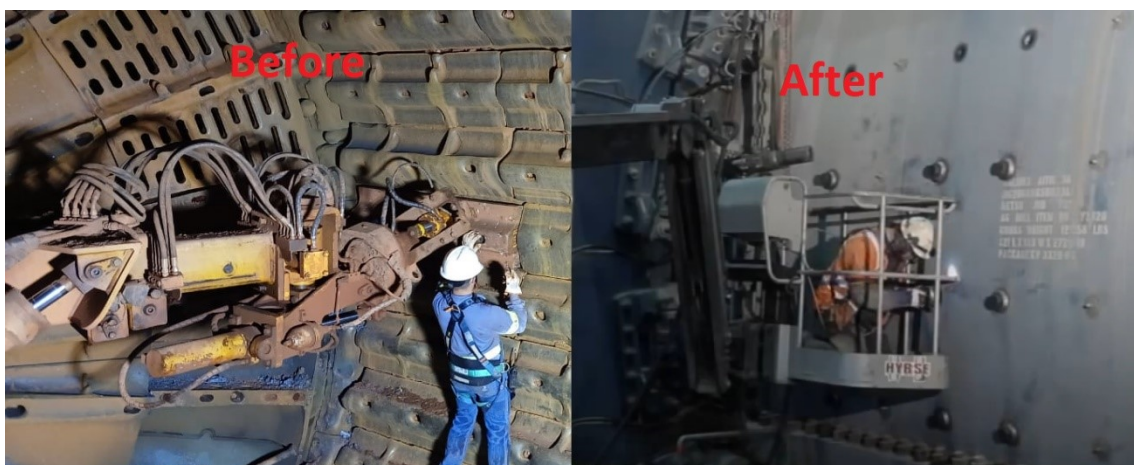
Figure 8. Before and after the improvement in linings
